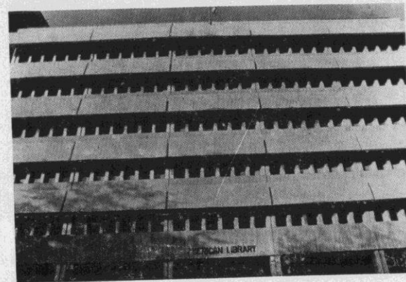
Fig. 48 American Library building in New Delhi shows details of sunshade projecting away from window to avoid transfer of heat into the interiors of building.
