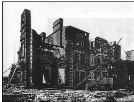
Halnaby Hall, Yorkshire, England, during demolition in 1952
